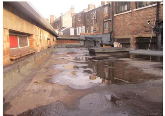
Photo 2 – Defective Flat Roof
